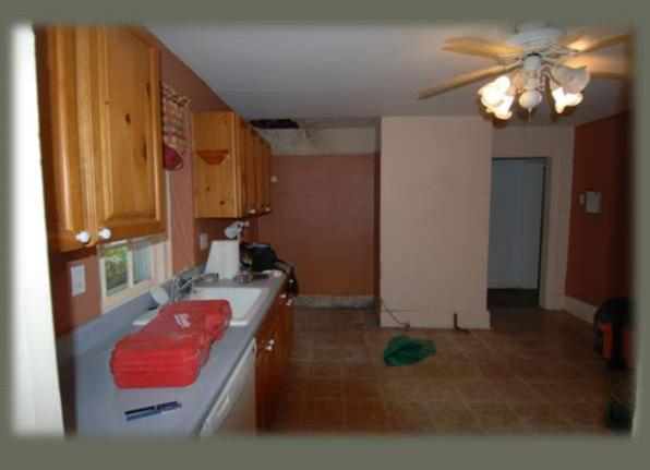
The refridgerater and stove have been moved the pantry walls removed, creating a more functional storage area in the corner of the kitchen.
